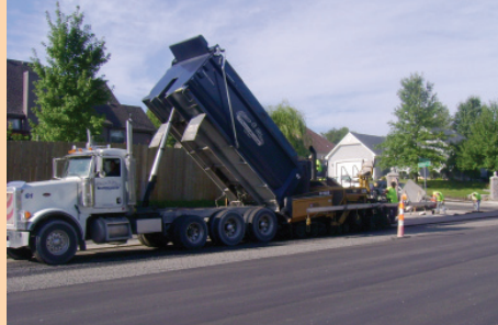
Crews working on R.D. Mize Road.
