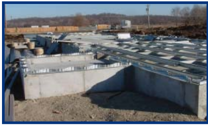
Construction is progressing at the Missouri 78 site.
